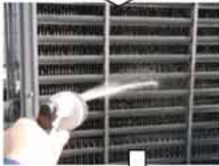
Water is hosed.
