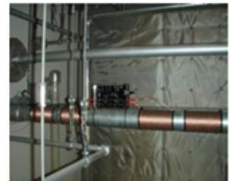
Used for the cooling towers C
