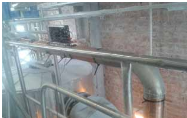
Installation of Vulcan S100 on lime kiln
