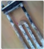
Heating element in a hot water tank
